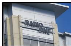
Radio One Headquarters Silver Spring, Maryland
